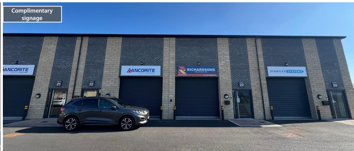
Plant room with 3-phase electric, DB board, water, solar control & BT fibre
